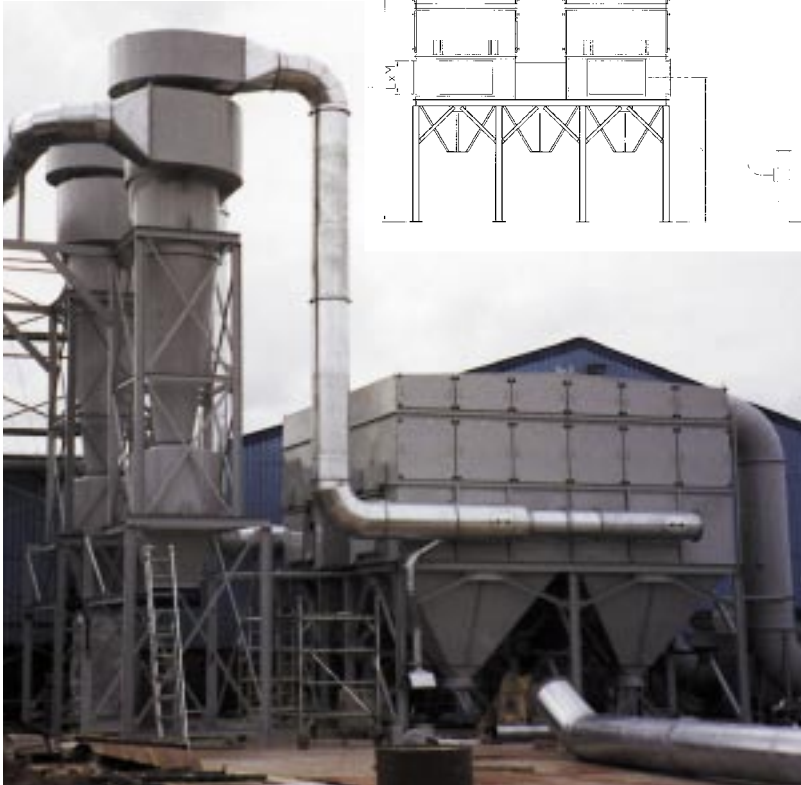
Valley Hopper – Large capacity filter units with Valley Hopper collection facility, mounted on supporting steelwork
